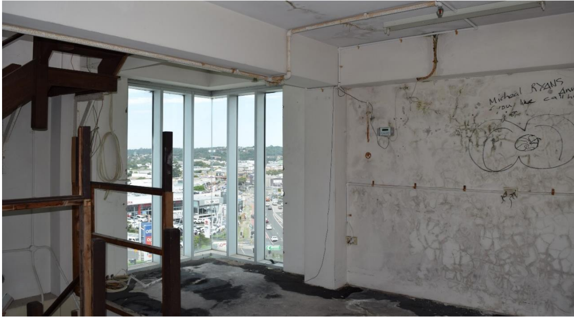
Figure 17: Looking towards the top-floor window within the clocktower. Note: Interior graffiti to the internal walls and rising/falling damp.
