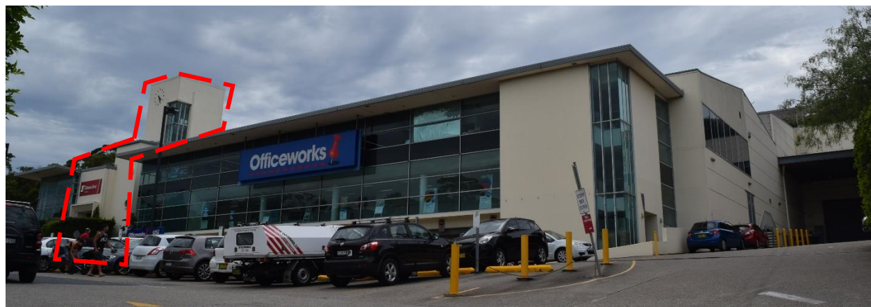
Figure 8: Looking northeast toward the western façade of the subject building within 800 Pittwater Road, from the south-west corner of the site. Note: The area identified as heritage fabric is indicated in red. Original fabric (building footprint) along the western elevation includes the structure below the glazing.
