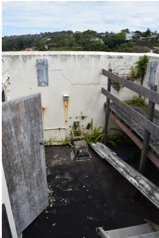
Figure 18: Image showing the condition of the roof-top of the clocktower including wooden platform and surface mounted conduits.
